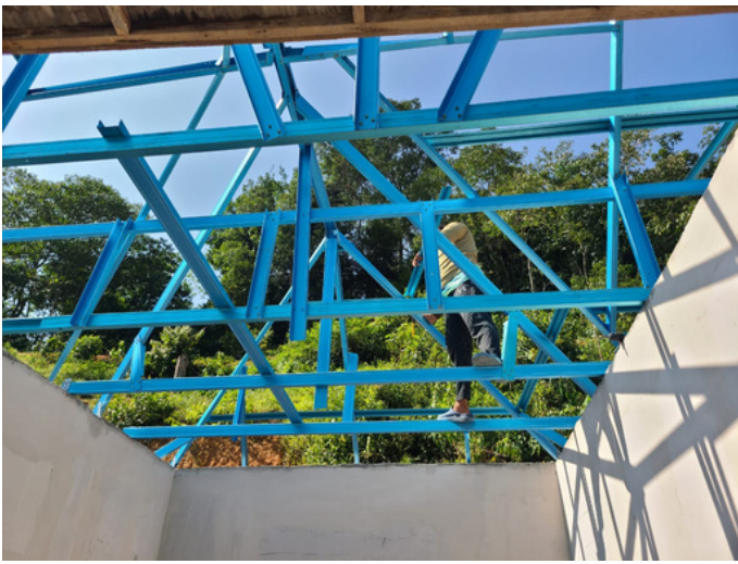
Installation of C-Channel
