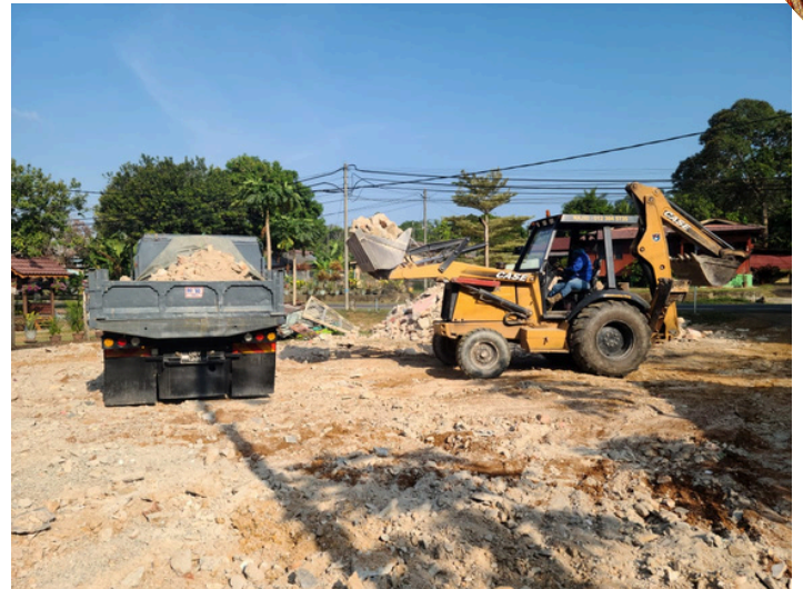
Loading of material waste
