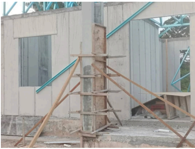
Pillar casting formwork
