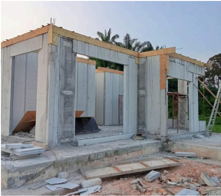
Roofbeam casting formwork
