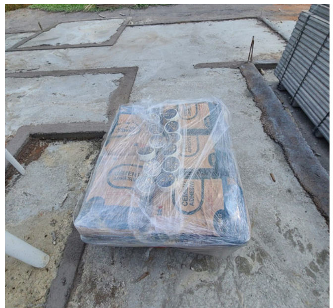
Delivery of construction material
