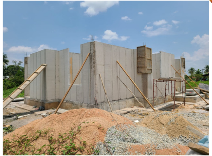
Finished installing WallPanel
