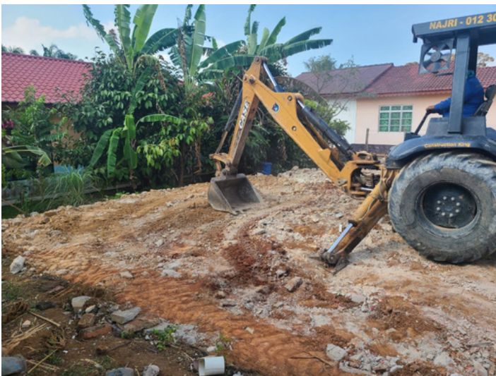
Ground levelling work
