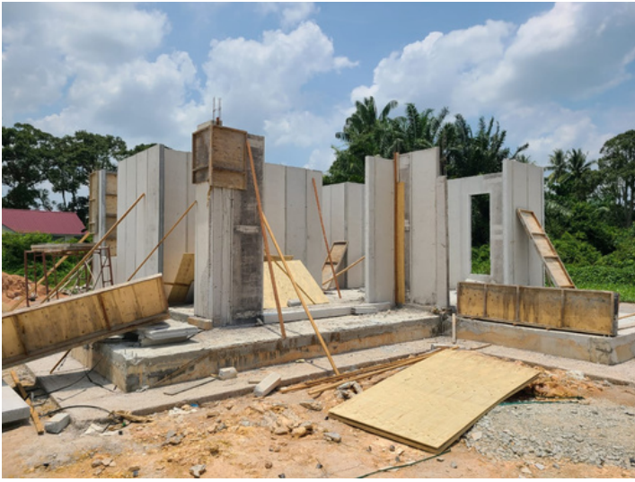
Installation of WallPanel
