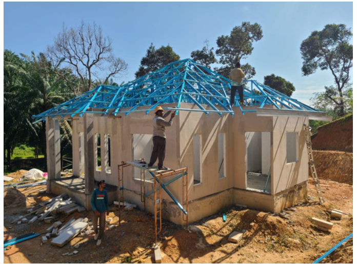
Roof trusses work
