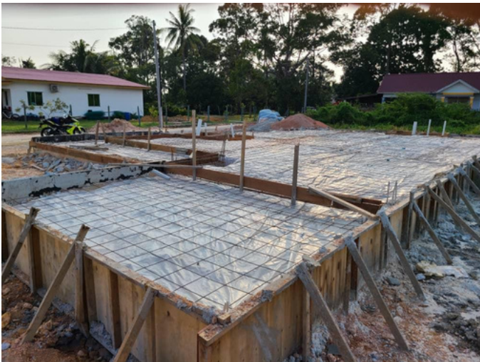
Finished foundation formwork
