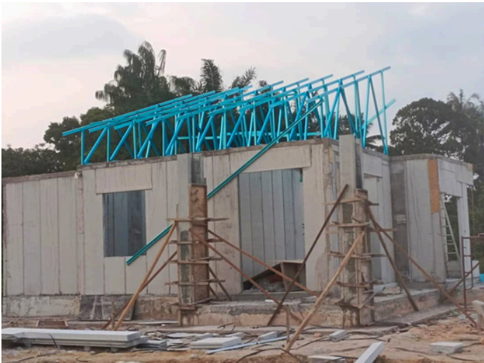
Installation of roof trusses
