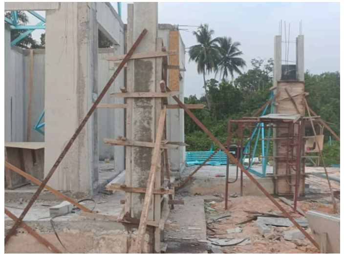
Pillar casting formwork
