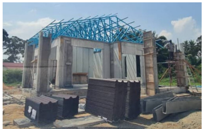
Finished installing roof trusses
