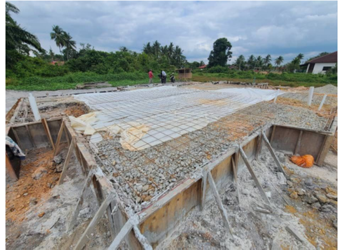
Installation of PE Sheet and BRC
