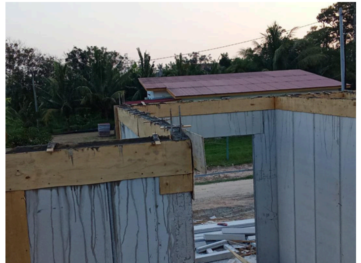
Roofbeam concrete work
