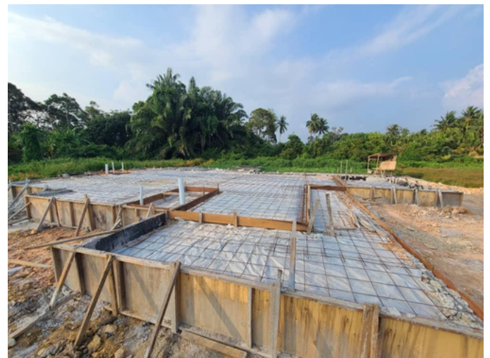
Finished foundation formwork
